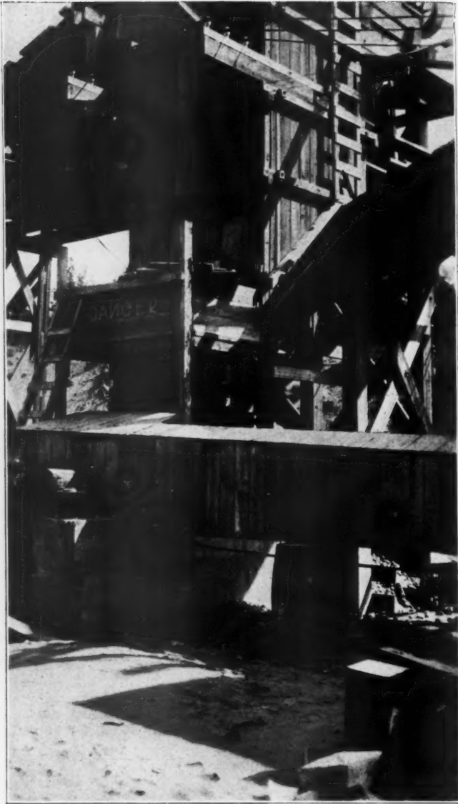
Structure for Supporting Scalping Screens With Crusher Below
